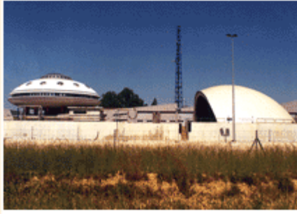
Deicing Salt Storage Choisey - France - 1998
