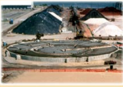
1. Ringbeam poured conventionally
