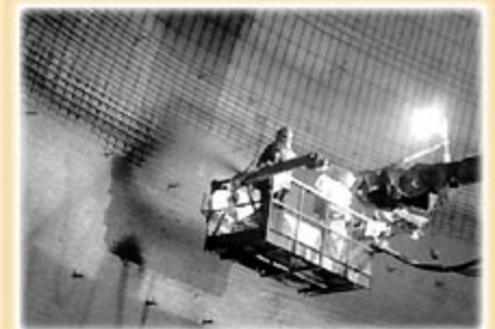
6. Concrete is spray applied on the steel grid.
