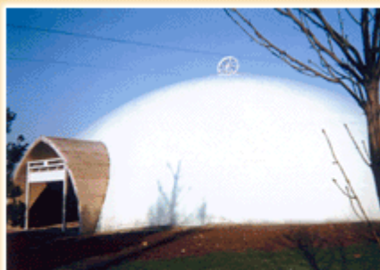
Cover for water treatment plant Height 13,50 m and diameter 40 m Houplin Ancoisne - France - 1992
