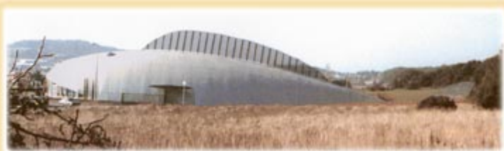
Public Aquarium length 72 m, maximum height 12 m, maximum width 30 m Cabries - France - 1999
