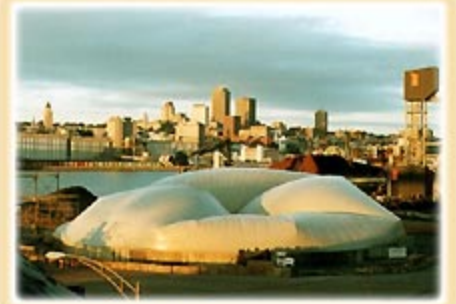
3. The airform is inflated and the pressure inside is stabilized.
